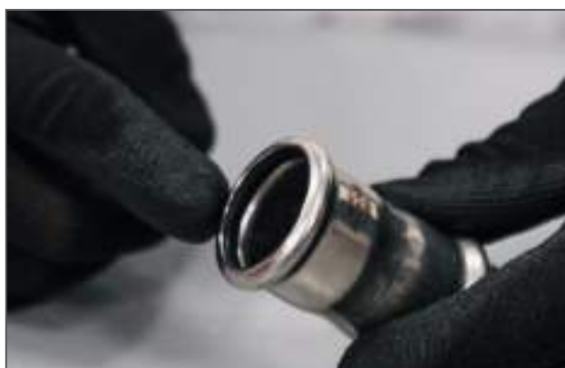
Controllo O-ring / Checking the sealing ring
